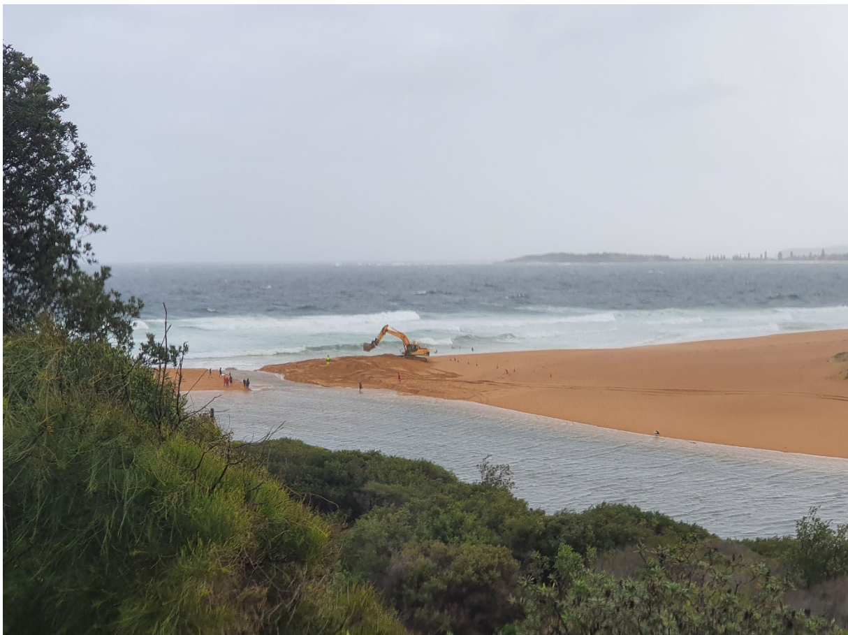
Figure 2.8 Mechanical opening of Narrabeen Lagoon entrance on 07 February 2020, 17:37 AEST (Source: Northern Beaches Council)
