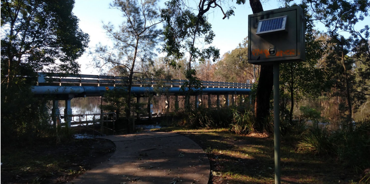
Walarah Creek at Wallarah Creek Bridge, 9:18 a.m. (AEDT) 11 February 2020 1.63 m AHD
