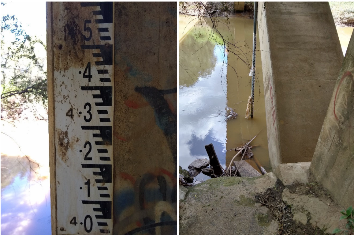
Prospect Creek at Lansdowne Bridge, 1:22 p.m. (AEDT) 19 February 2020 (post flood)
