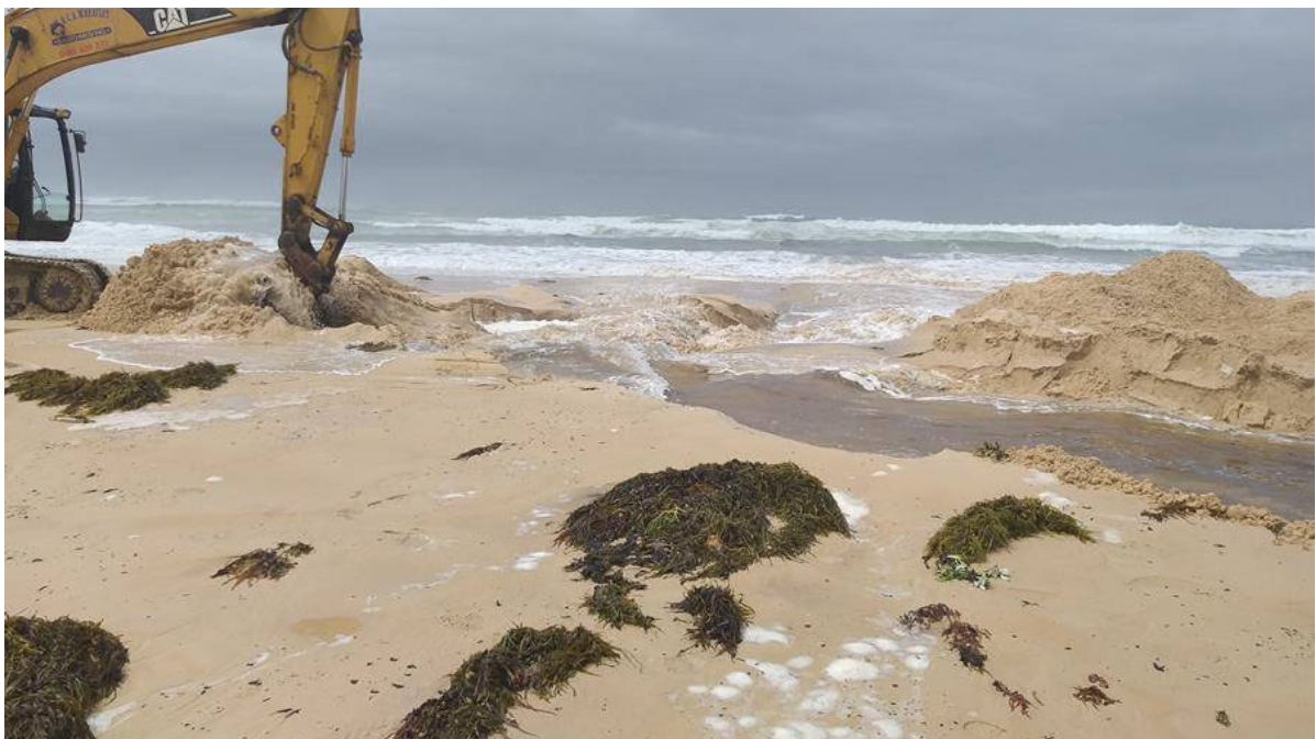
Figure 2.11 Mechanical opening of Lake Conjola entrance on 10 February 2020
