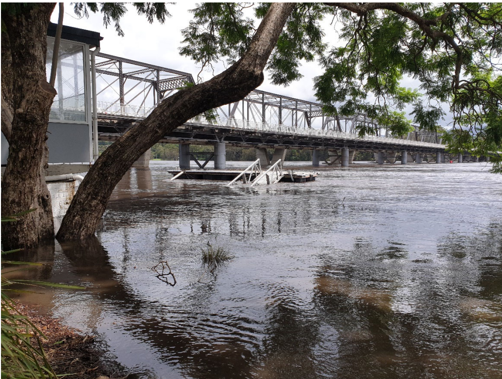
Shoalhaven River at Nowra Bridge, 12:22 p.m. (AEDT) 10 February 2020 3.64 m AHD
